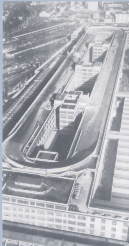
Fiat's five-story factory, built in the 1920s, features a rooftop test track.
